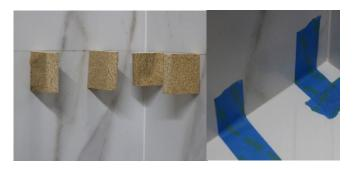
Place a piece of masking tape on top of support block, so that sealant does not prevent removal of support blocks after cured.
