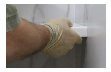
Avoid large gaps between the Wetwall surface and corner shelf by sanding. or cutting to ensure good fit to wall panels. Apply wooden support blocks (4) with hot melt to under location where corner shelf is to be mounted.
