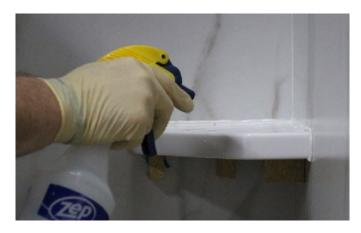
Secure the corner shelf in place with tape. Allow 24 hours for the sealant to dry before use and remove support blocks by gently tapping them loose from Wetwall panel.
