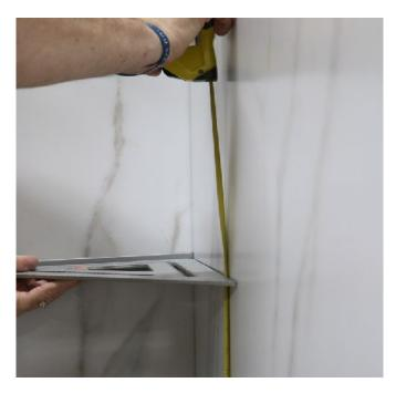
Using a level, mark location where corner shelf is to be installed on the Wetwall panels. (Recommend the Corner Shelf would be installed 43" from the shower floor).
