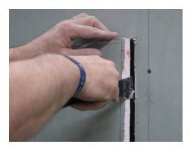
Cut and remove the current substrate to expose the wall structural framing.
