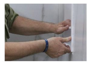
Secure the niche in place with tape. Allow 24 hours for the sealant to dry before use.
